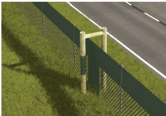
Figure H3 Escape pole with H-shaped design offering resting bar and safe refuge from the ground. This design was trialled during this study
